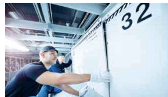
Installation of a replacement lining panel
