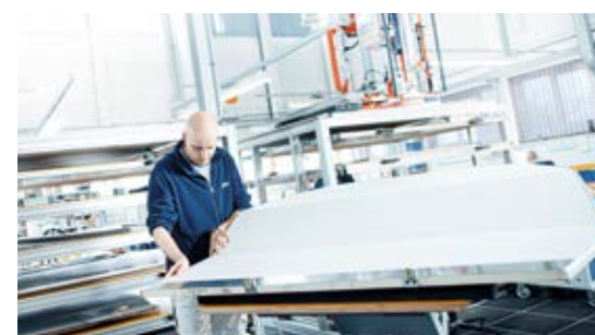
Quality-conscious completion of a partition wall
