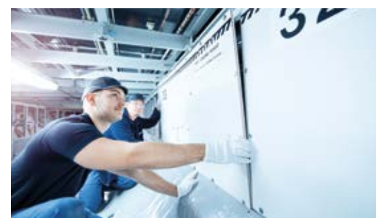
Installation of a replacement lining panel
